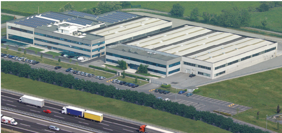
The headquarter of Maico Italia Spa, Lonato del Garda (Brescia), Italy
